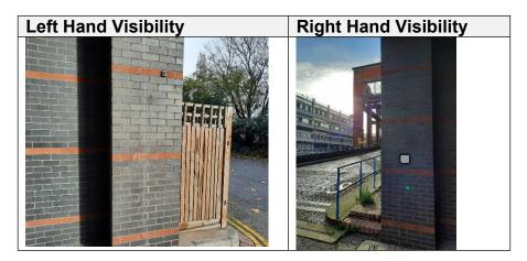
The northern access junction (egress) has been designed as the site egress with a no-entry sign and the building line angled to allow right hand visibility towards vehicles approaching from Observatory Car Park and car parks to the rear of the High Street Shops. A fence appears to have been erected which would need to be removed/reduced to allow suitable visibility.
